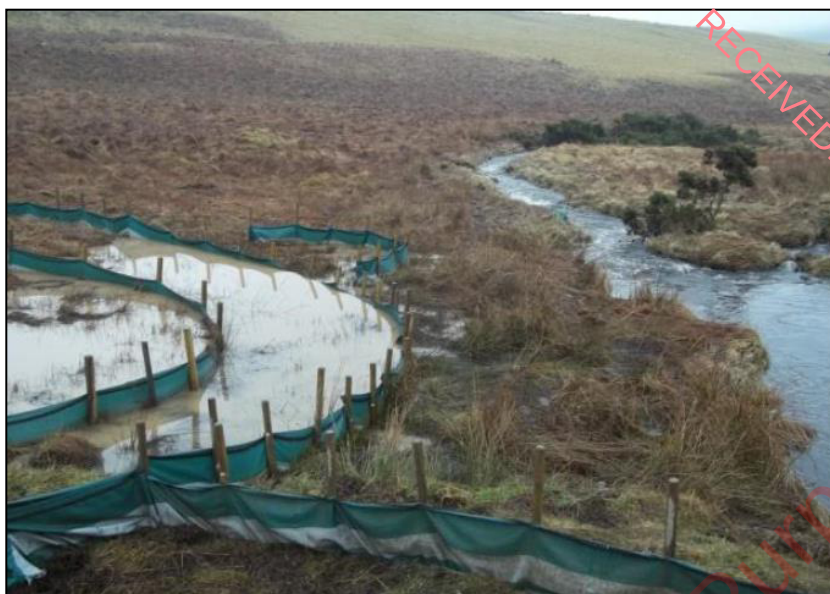
Plate 5.1: Photograph of Silt Fencing
