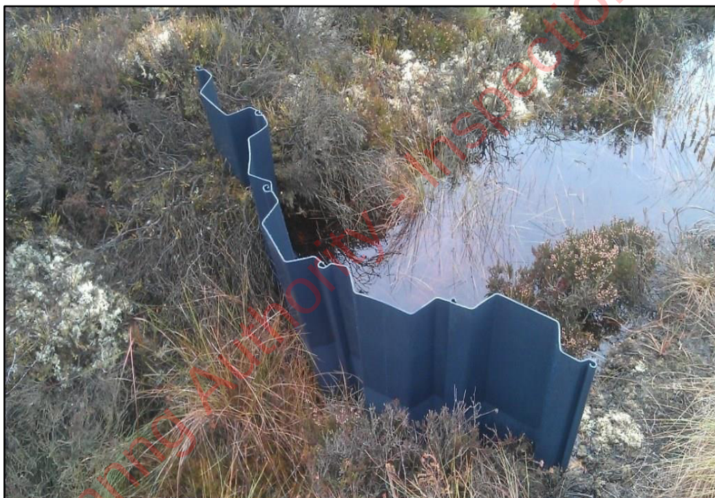
Plate 3. An example of a recycled plastic dam used to block functioning drains on a raised bog site.
